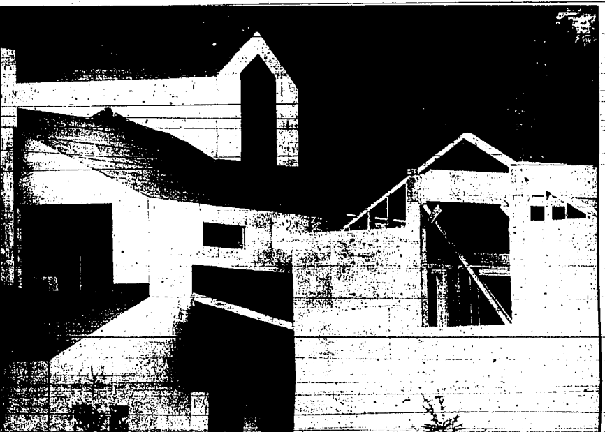
Structures are on the rise in the Wood River Valley as building permits are up about 50 percent from last year. Times-News photo/TERESA TAMURA
