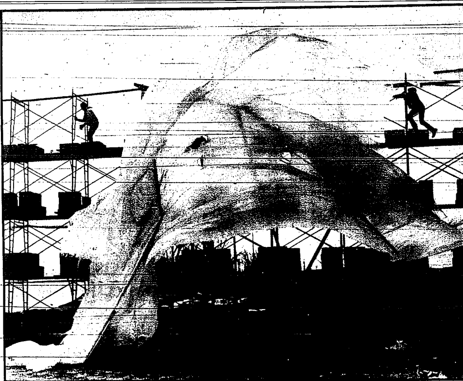
Construction workers John Mullins, left, and Bill Korsen battle mother nature as wind plays havoc with the Sears construction site
