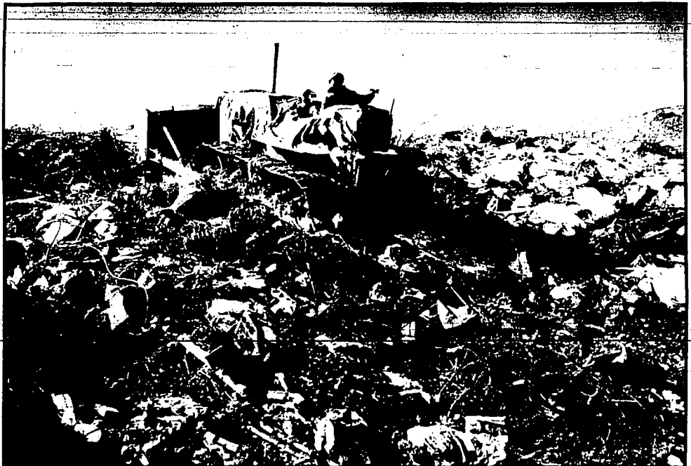
At Twin Falls, County's main landfill diapers, along with other refuse brought in, are compacted by bulldozer before being buried
