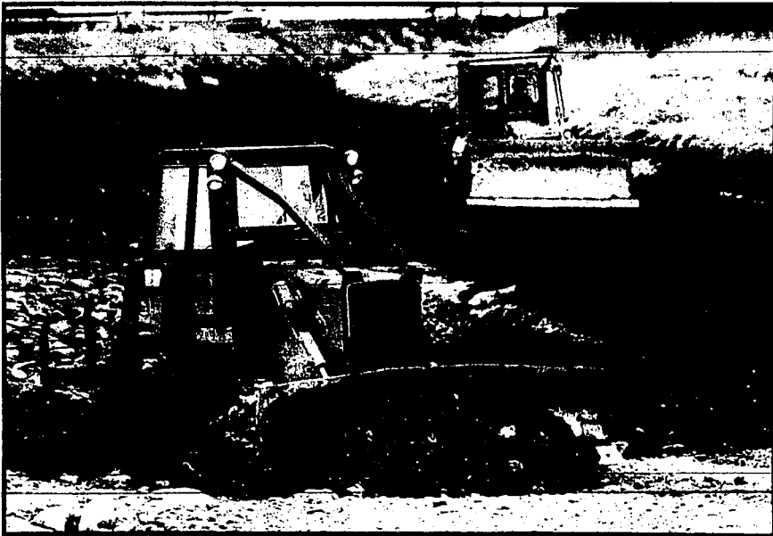
Bulldozers level the bottom of the Highline Canal near South Blue Lakes Boulevard as part of regular maintenance
