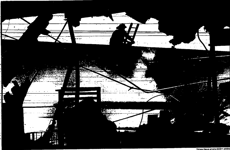
A Jerome firefighter hoses down the charred remains of the Volco building, which was gutted Friday morning by fire
