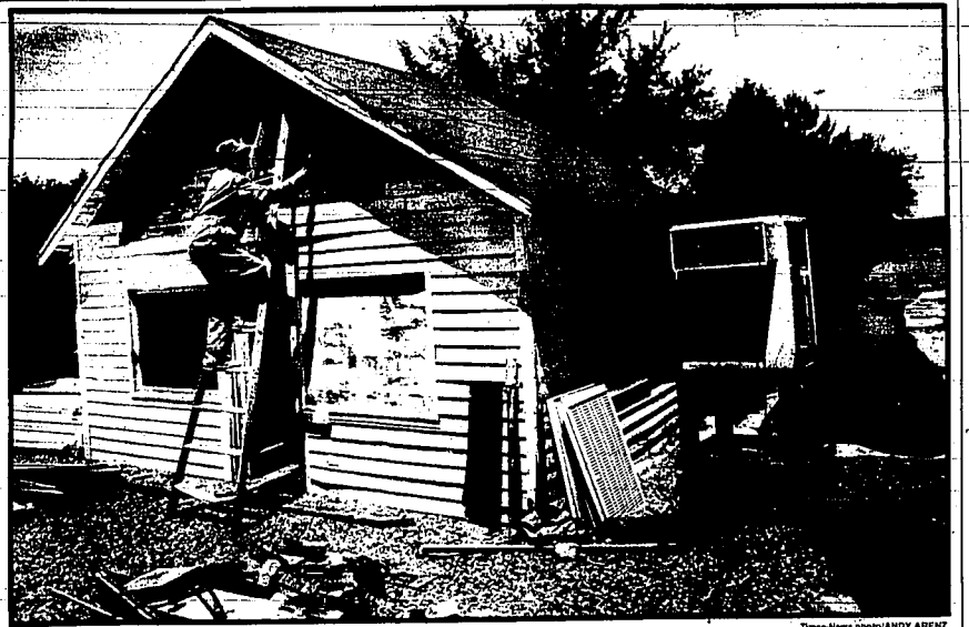
Marvin Fisher, Hansen, drafts apart a shed that was damaged by the April flood that followed the canal at right
