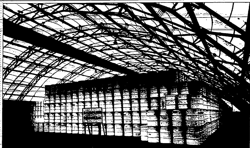
Since 1980, transuranic waste has been stored in inflatable plastic buildings
