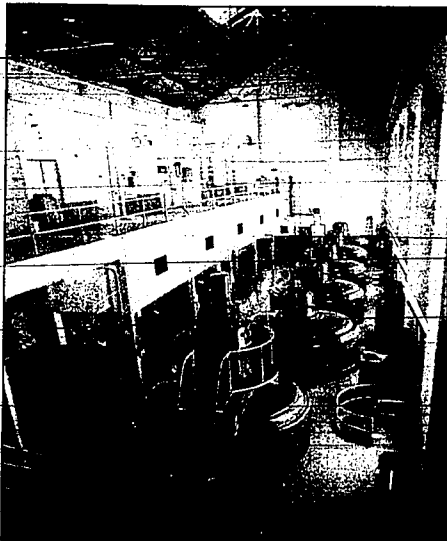
Six of the seven generators and turbines in the historic Minidoka Dam powerhouse are scheduled for replacement
