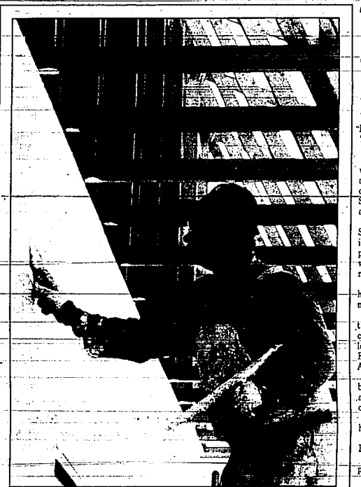
Finishing touches Under a wood framed canopy Larry McBride smoothes out the walls of Centennial Square, the strip mall being built on Blue Lakes Boulevard North.
