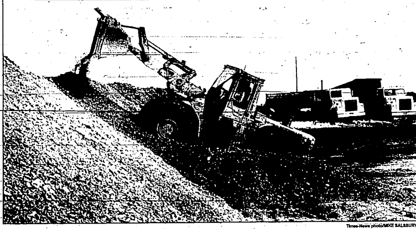
Gravel is stacked after being unloaded by workers Tuesday afternoon. It will be used as fill for the Milner Dam project.
