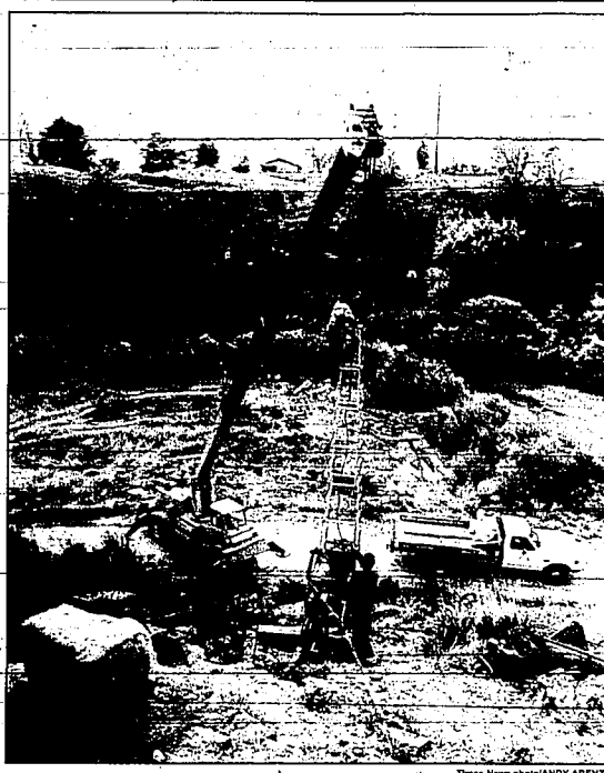
Workers assemble a core drill in Rock Creek Canyon at the Victory Bridge site. Times-News photo/ANDY ARENZ
