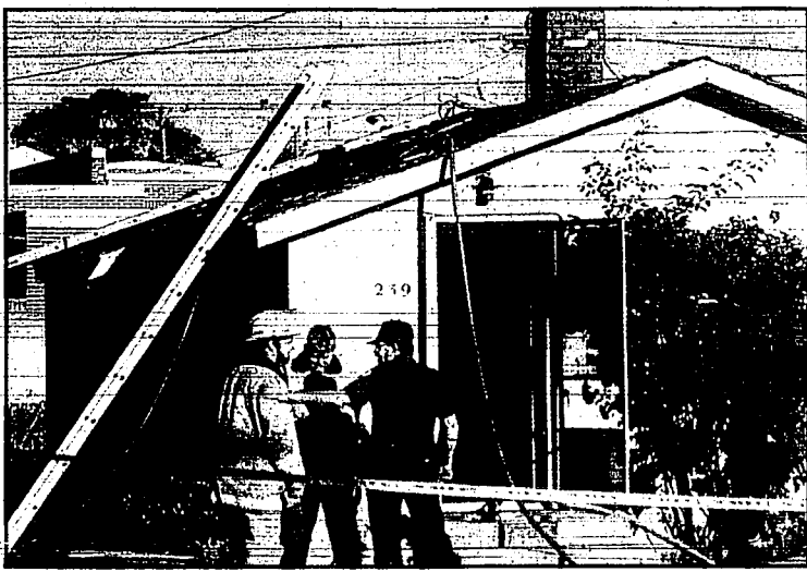
Emergency workers pause outside the location of Tuesday's fatal fire. Frank Earl Taylor died in the blaze as the back portion of the Kimberly home was burned extensively.
