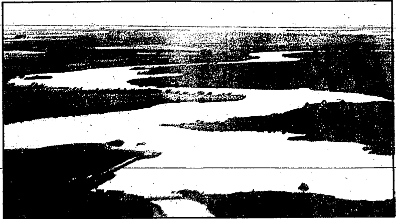
The water diverted at Milner Dam irrigates much of the Magic Valley's farmland. Hydro power plants are under construction at the dam and downstream.
