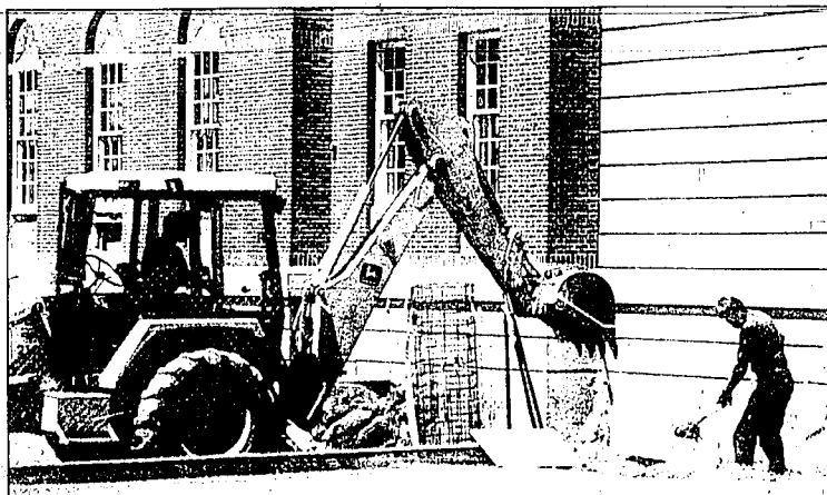
Bryan Hemenway scoops up a shovelful of dirt while Mark Rowley in the backhoe operates a bigger shovel at the Twin Falls Public Library addition site Thursday. Construction has begun on the expansion, which will double the size of the library.
