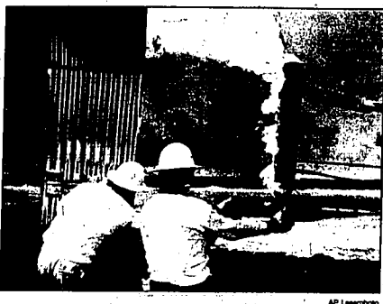
Larry Nixon, of Spring, Texas, holds a tin shield to deflect heat while Ace Barnes of Odessa, Texas, directs the boom operator in efforts to put out a burning well in Greater Burgan Oil Field.
