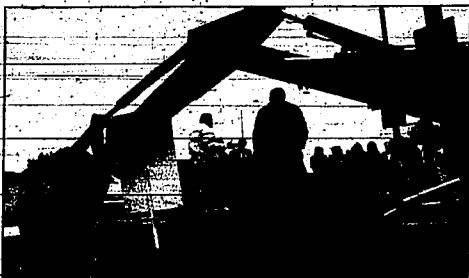
ANDY ARENZ/The Times-News The voluntary beautification project was officially started Friday with a hole broken through the asphalt beside the Chamber of Commerce building.
