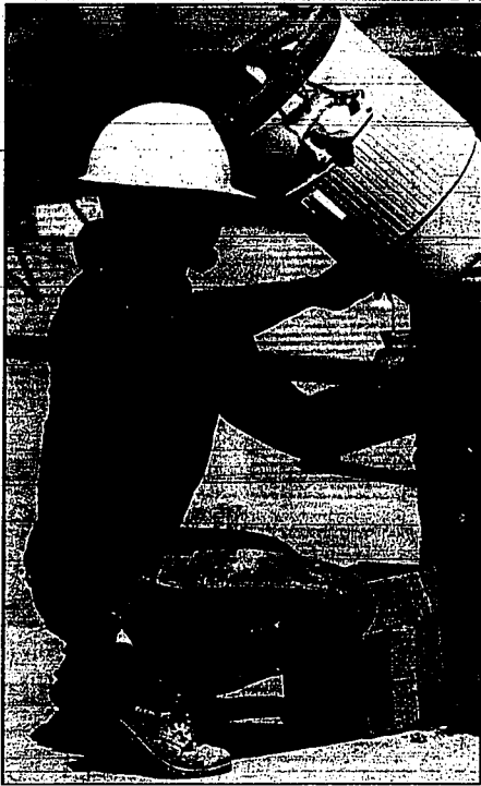
Eddie Jaramillo takes a water break after laying blocks on CSI's agriculture science center where temperatures reached an unofficial 102 degrees.
