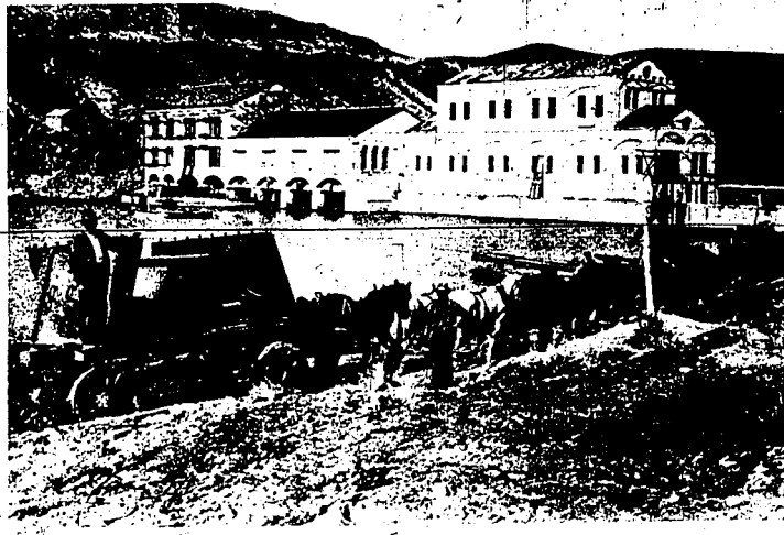
Construction of Swan Falls Hydroelectric Plant
