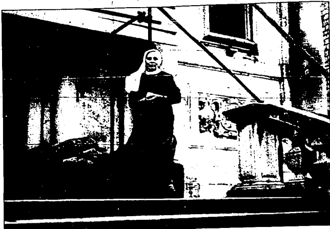
A nun stands before scaffolding and sandbags used to help protect St. Vlaho church in Dubrovnik during the Yugoslavian army's three-week siege of the historic Croatian port city.
