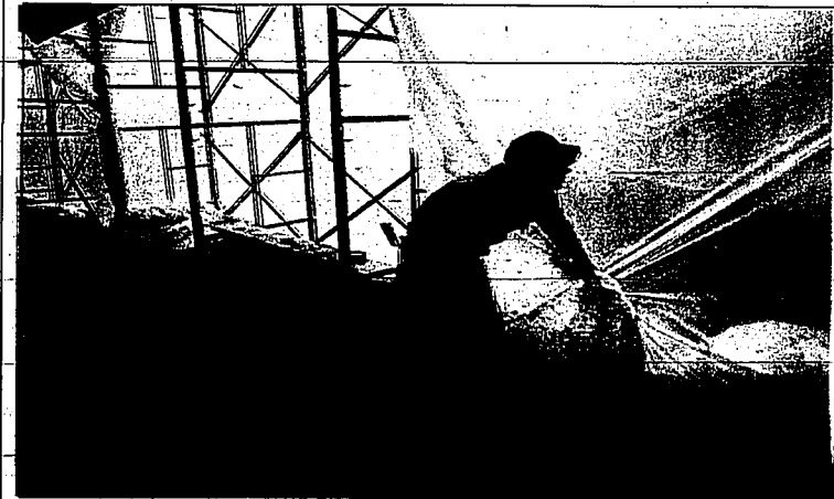
Working in a bubble-like environment is fine for Dave Taylor, preparing to coat a house with an exterior finishing. The partner in T.J. Exteriors said applying the coating requires a minimum temperature of 40 degrees and without the help of mother nature the crew has to create its own warm weather using plastic sheeting and gas heaters. Covering this two-story house on Candlewood Circle in Twin Falls took an entire work day, according to Taylor.
