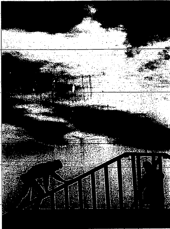
Carpenters Mark Donning, left, and Larry Cossey set a truss on a house under the afternoon sky in Twin Falls. Cossey said the weather was "great" Tuesday for construction work as the sun warmed the air to 42 degrees in town. The house they are building is the first of 22 units planned for the Green Tree Estates by Willis Inc. on Cypress Way.
