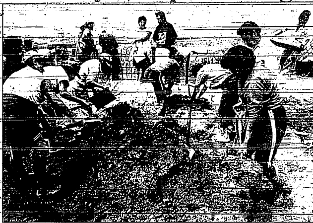
Women make mud bricks to build a health center in Villa El Salvador, Peru, last week.
