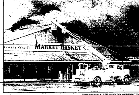
A short-circuit in wiring along the store's ceiling likely sparked Tuesday's fire, officials determined Thursday. The store, whose slogan is, "If we don't have it, you don't need it," was an important part of the community, he said. Although there are convenience stores in
