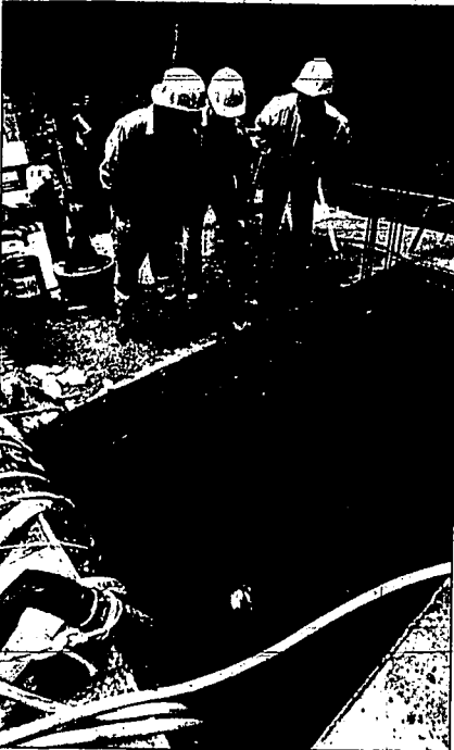
Utility workers in Chicago check water levels in the bottom of a utility sub-station Tuesday where water leaked during flooding.
