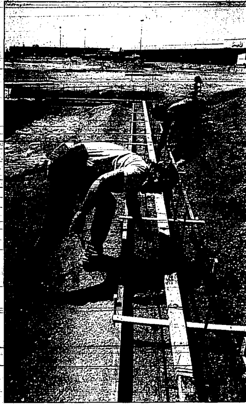
Roger Shaddy, front, and Fred Hernandez prepare footing forms at the Campbell Homes nursing care complex project.
