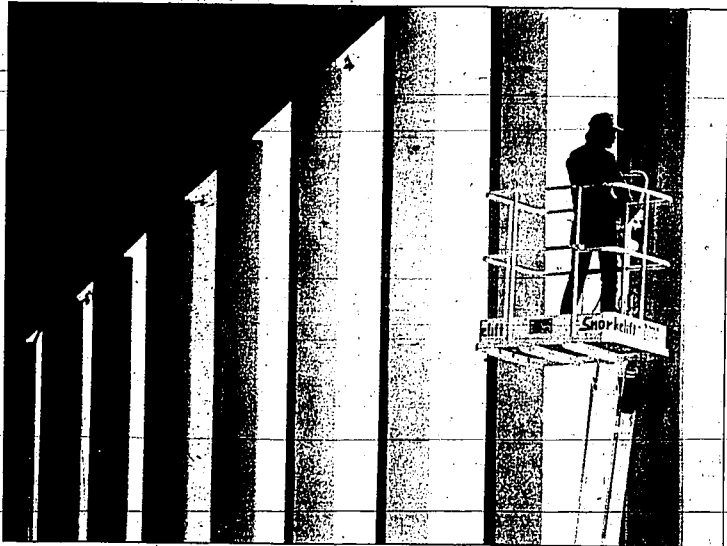
Framed within a row of beams at the Twin Falls County Fairgrounds, Al Woolstenhulme of Burley makes his way to the ground. Workers were busy Wednesday installing iron beams for additional support to the fair's grandstand.
