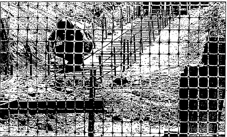
Patterns of girth frame construction worker Ron Moore as he provides labor for the new expansion project at Norco Windows on Thursday. Workers have started constructing the foundation of a new receiving building at the site.
