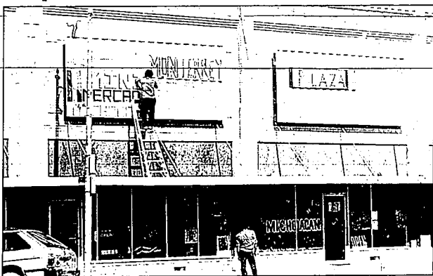
Workers repair a sign above the Monterey Plaza store that sells Hispanic food and merchandise in downtown Rupert recently.
