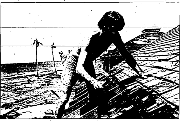
John Hunt hammers in exposed nails on the heavily-damaged roof of a friend's house in Poipu on Kauai.
