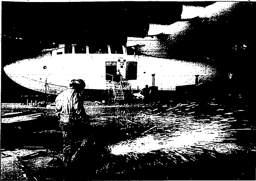
Workers begin the process of sectioning the historic HK-1 Hughes Flying Boat, built by the late Howard Hughes, Monday in Long Beach, Calif. The Flying Boat, known as The Spruce Goose, will be cut up into 38 separate elements for transportation by land and sea to its new home at the Evergreen AirVenture Museum in McMinnville, Ore.
