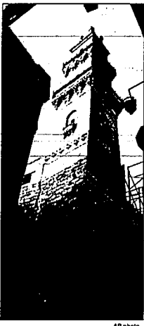
Wednesday's earthquake left a crack in the el-Ghouri Mosque, one of about 30 seriously damaged in Cairo.
