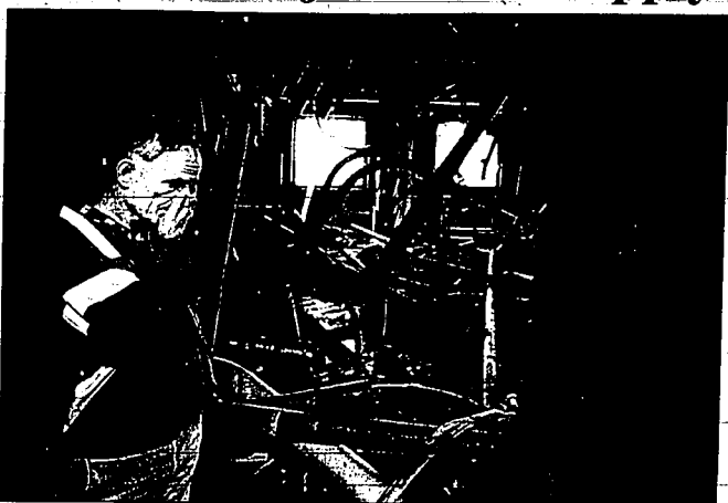
AP photo A worker surveys the damage done to Sarajevo's flour mill Monday. The mill, which makes more than 90 percent of Sarajevo's bread and pasta, was damaged Sunday during heavy shelling.
