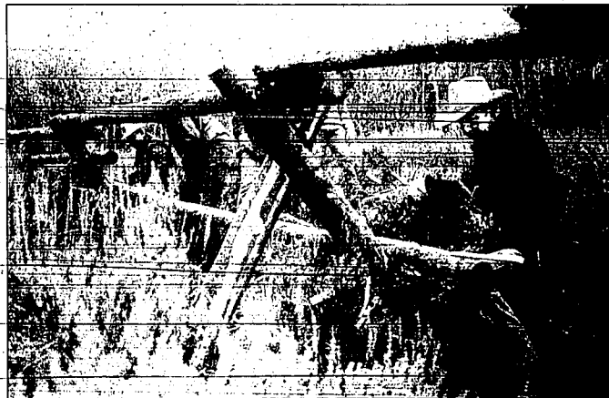
Lee Kocmick fits a fence pole to the upright buck.
