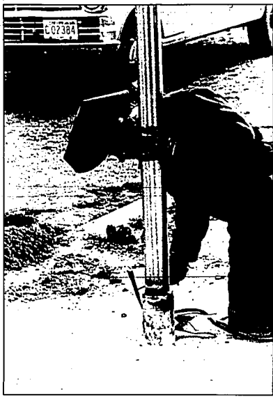
Tom Driese of Burley welds a support for a basketball hoop at an outside court being completed at Big Valley School in Rupert.
