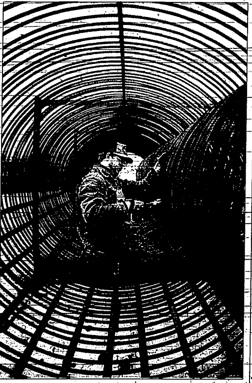
In a web of steel reinforcing bars, construction worker Kent Bateman fastens the metal hoops into a pier column frame for the Singing Bridge replacement. When completed, the bridge will carry Shoshone Street across Rock Creek Canyon in Twin Falls.
