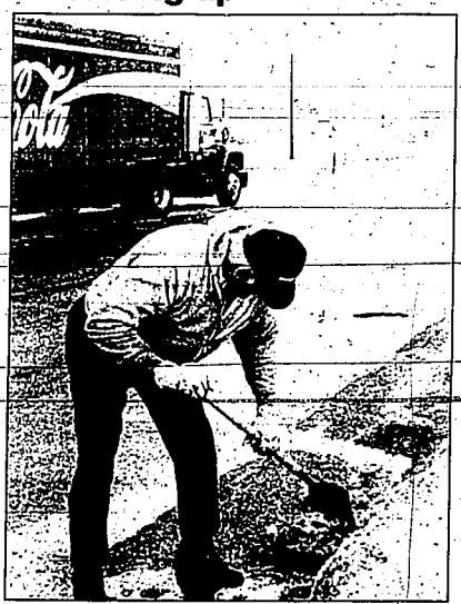
Heyburn city employee Joe Thomson removes ice from around a storm drain along Highway 30 Wednesday. In order to locate the ice-covered drain, he first used a metal detector.
