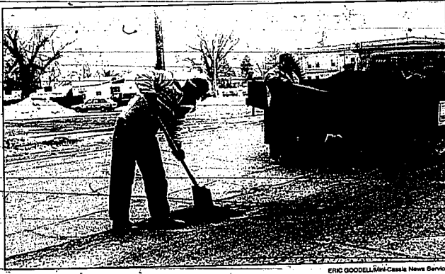
Rupert city employees Doug Bruno, left, and Terry Tracy fill in pot-holes along Eighth Street after moisture this winter caused extensive damage to Mini-Cassia roads.
