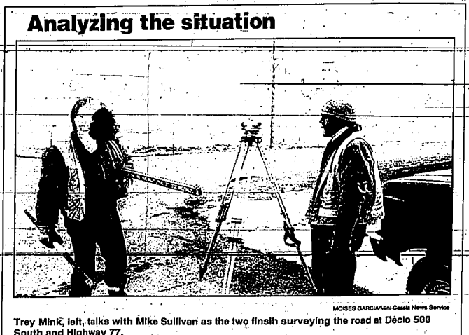
Troy Mink, left, talks with Mike Sullivan as the two finish surveying the road at Déclo 500 South and Highway 77.
