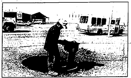
Duane Earl of Earl's Roofing fixes a pothole in Rupert.
