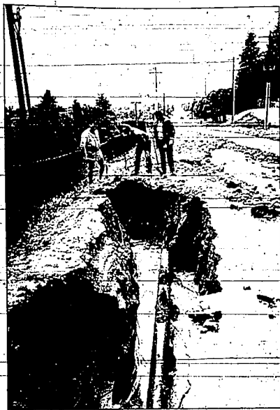
Residents check flooding damage along a rural street near East Wenatchee, Wash., Monday. Over two inches of rain damaged about 100 homes and many roads Monday afternoon.
