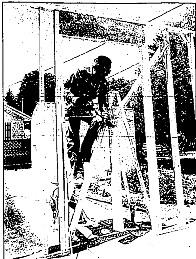
ERIC GOODSELL/Mini-Cassia News Service Cal Sterling of Burley works constructing a garage in Rupert Thursday.
