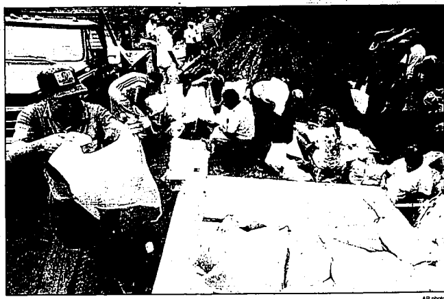
Iowa farmer Crafton Meeker hoists a sandbag into a pickup Tuesday in Oquawka, Ill. Volunteers filled the bags for use along an eroded section of the Henderson Creek levee about two miles east of that trouble spot on the Mississippi River.
