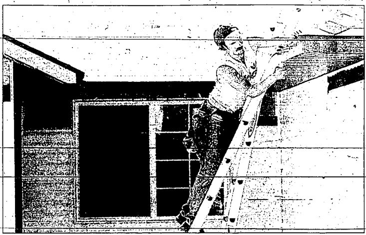
Greg Ayers of Northwest Specialties Inc. installs siding to a new home in Twin Falls where building activity is at record pace.
