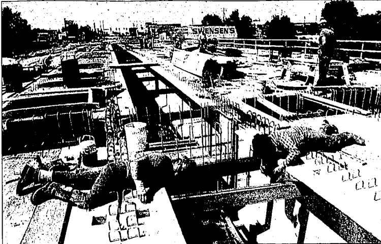
Workers are busy and running on schedule on the replacement for Twin Falls Singing Bridge, set to be finished in October. Despite harsh weather, construction company official Gaylord Hudson said, 'We might beat the deadline.'
