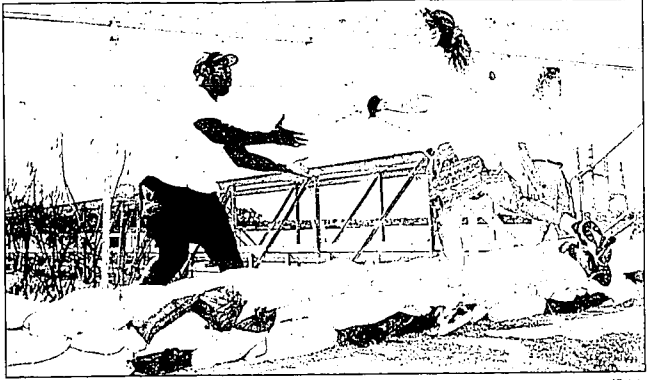
Clark Oil Co. employees work against the clock Thursday to build a sandbag levee around gas storage tanks in St. Louis. The Mississippi River is expected to crest at 48 feet Tuesday.
