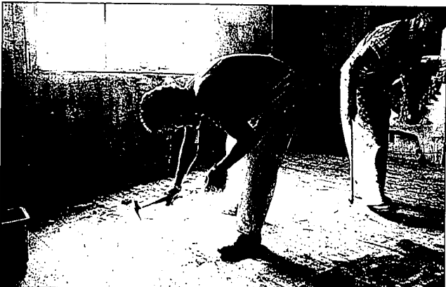
Canadian volunteers work Friday in Des Moines, Iowa, to repair a flood-damaged home. A busload of Canadians is helping Des Moines residents as part of a project called Hands Across the Border.
