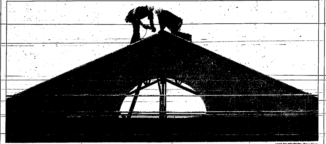
Steelworkers John Williams, left, and Richard Satterjee combine efforts Monday afternoon while working on the construction of a decorative roof section at the new Wilson-Bates building on Pole Line Road in Twin Falls. Work at the site has been going on for about three months, with a grand opening scheduled for Sept. 15.
