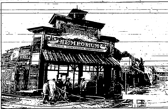
Firemen begin their cleanup Saturday after a huge fire roared through several businesses in downtown Winthrop, Wash., Friday evening. The fire apparently started in the basement of the Tender Foot, a grocery store on the main road through Winthrop.
