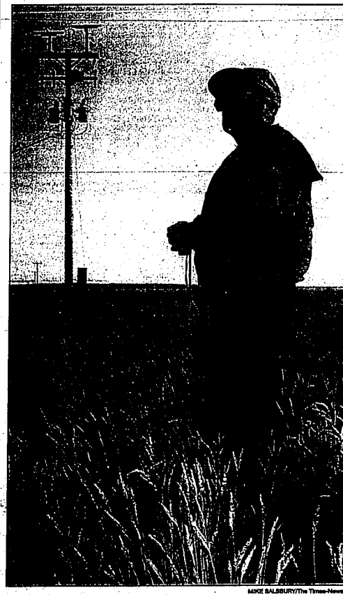
After a golden eagle brought a piece of barbed wire into a power pole nest, electrocuting its young, Idaho Power Co. installed perches atop this pole and above high-voltage lines, according to company engineer Lee Bunch. A Monday examination of the site showed eagles have been using the perches, Bunch said.
