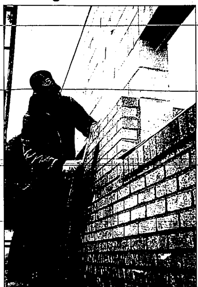
Marvin Cannell lays bricks on an addition to the Idaho Mill and Industrial Supply in Burley.
